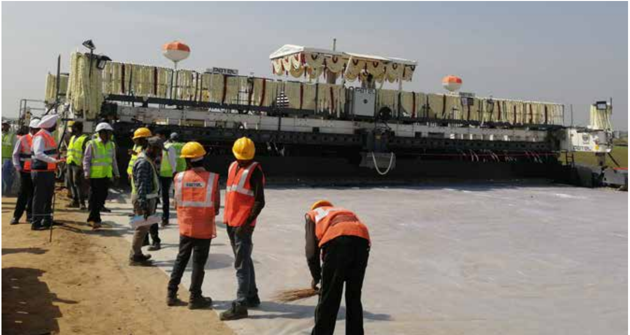
The SP-1600 fully automatic slip-form concrete paver from Wirtgen has a full paving width of 18.75 m.
